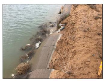
PHOTO: A portion of the deteriorated water canal at the Navajo Indian Irrigation Project.
