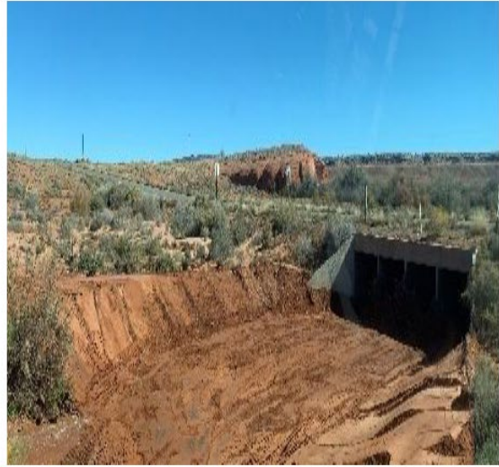
AFTER – N63 CBC cleanout and fence repair.
