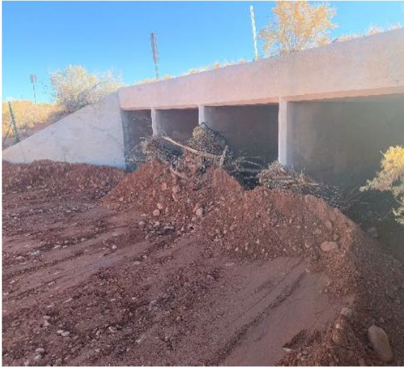
DURING – N63 CBC Cleanout and fence repair.
