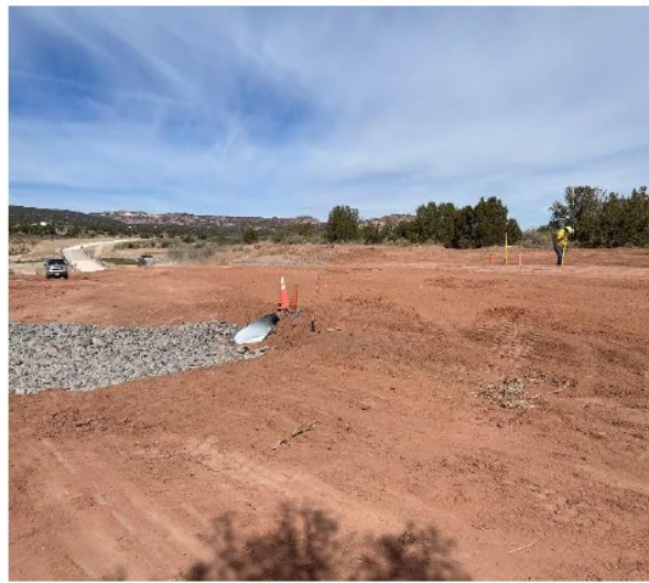
AFTER – Outlet protection.
