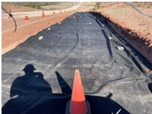
DURING – Assist Ft. Defiance w/ erosion control installation utilizing placed riprap material.
