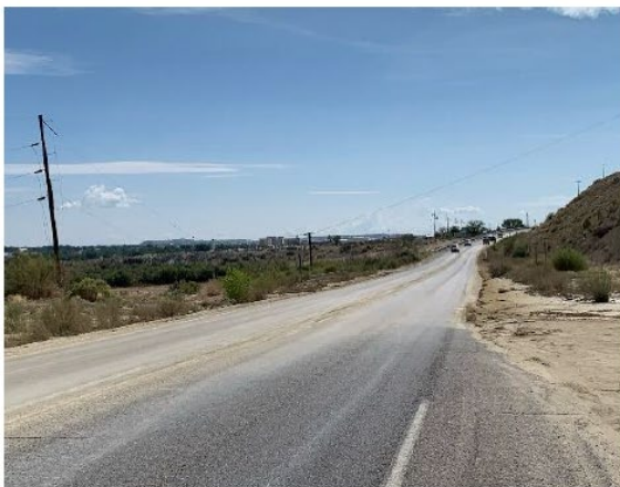
Monsoon 2021 – Route N36 silt accumulation along roadway was removed to reestablish ditch line and fence repairs.
