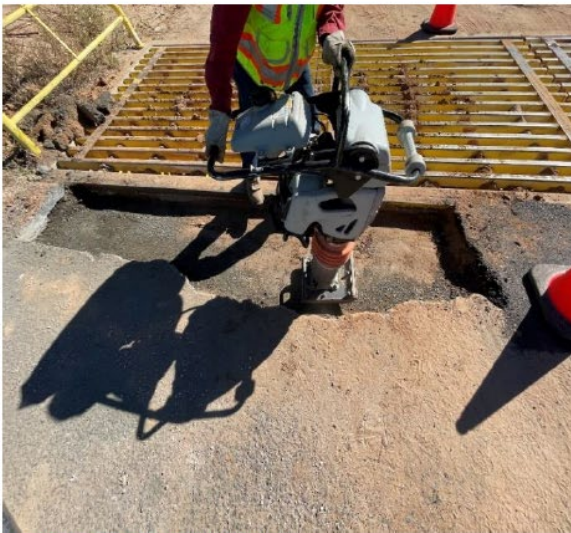
DURING – Cattleguard repairs.
