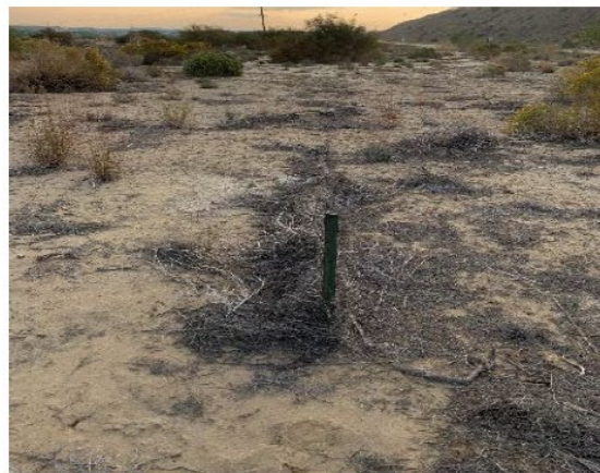
Monsoon 2021 – Route N36 silt accumulation along roadway was removed to reestablish ditch line and fence repairs.
