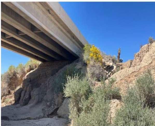
Bridge N533 West Abutment Erosion Bridge N533
