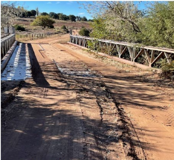
BEFORE – Prior to bridge wooden planks replacement.
