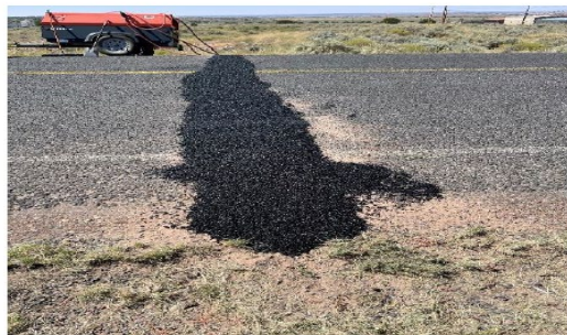
DURING – Roadway surface repaired using UPM.
