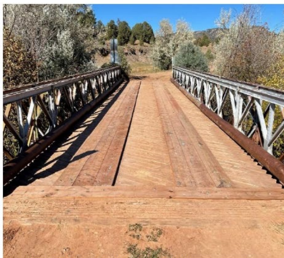
AFTER – Replaced wooden bridge planks.
