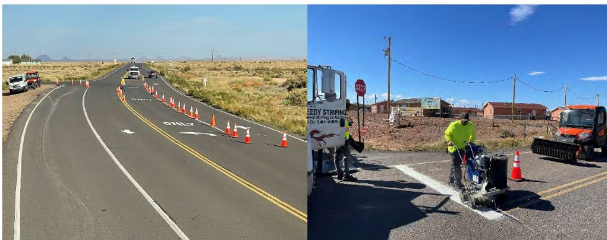
Contractor placing thermoplastic paint on roadway within Western Agency.
