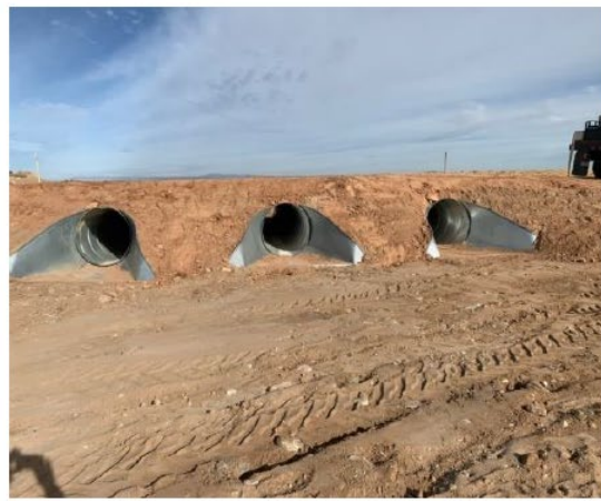
AFTER – N5113 New pipe installation. Roadway reopened.
