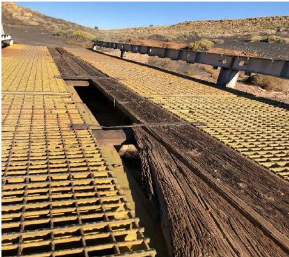
BEFORE - Bridge N319 – Damaged bridge deck.
