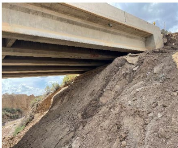
West Abutment Erosion Repair
