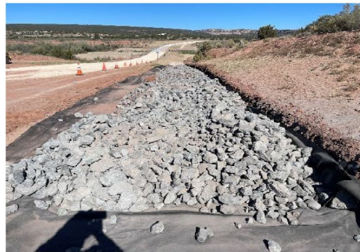
DURING – Assist Ft. Defiance w/ erosion control installation utilizing placed riprap material.
