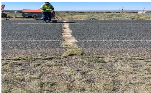
BEFORE – New Lands Road: Pavement cracks
